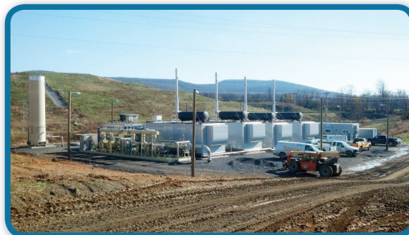
Landfill Gas Plant under Final Construction 2012
