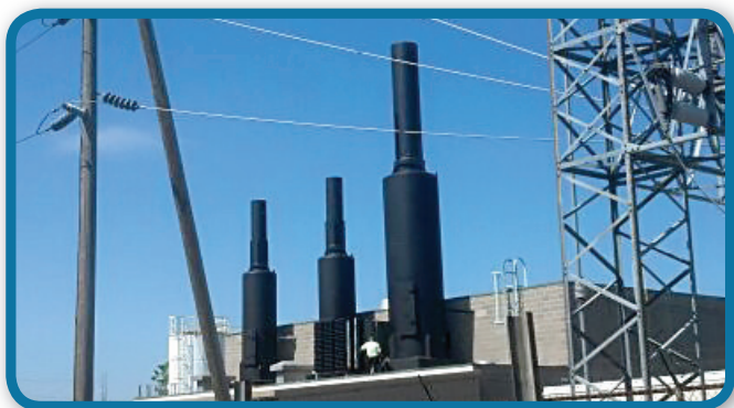
The FSGS is located on and visible from Grant Street
